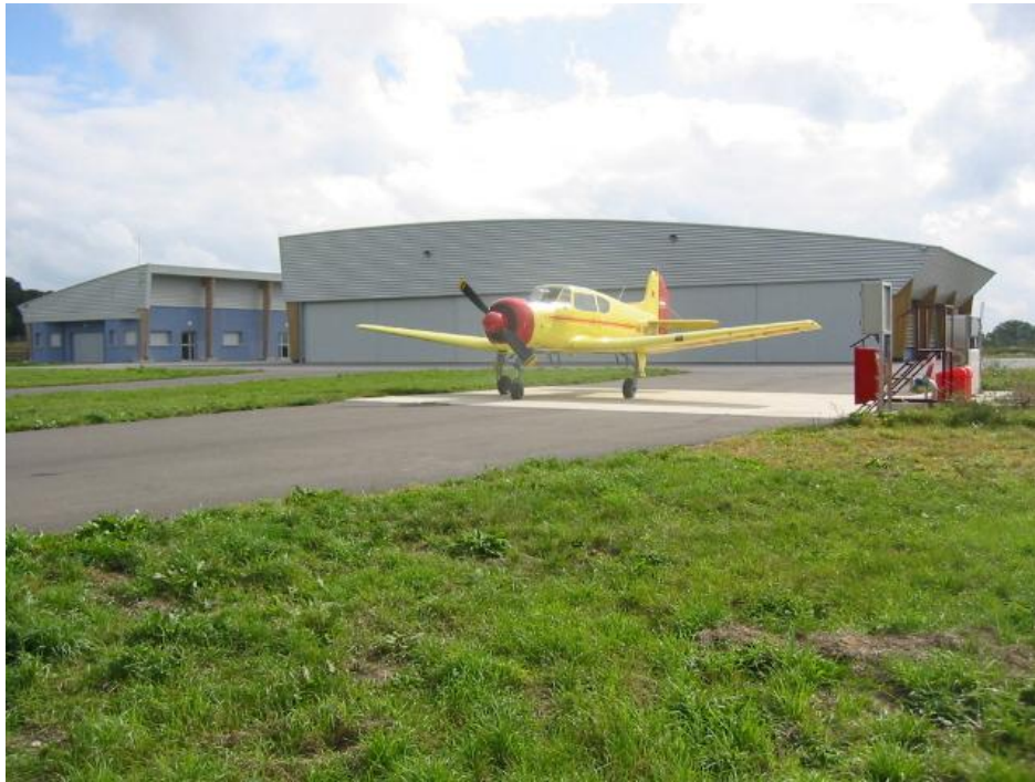
At Mortagne with beautifully designed hangars and offices behind
